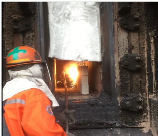
Fig.2. B6 insulation bricks where ceramic welding was carried out in the coke oven chamber.
